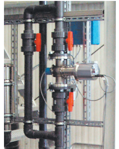
Straight pipe installation with ultrasonic cleaning system
